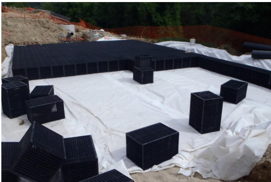
**FIGURA 9:** DEPÓSITO RETICULAR INSTALADO EN GUERENDIAIN (NAVARRA).
