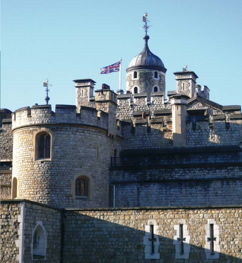
Several World Heritage sites are threatened by tidal flooding in the City of London (United Kingdom), here: the Tower of London.
