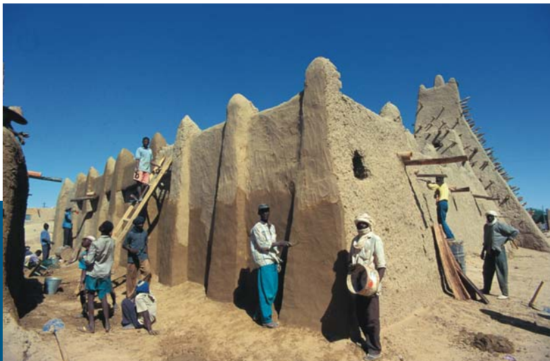
The restoration of the ancient mosques of Timbuktu was carried out by local craftsmen using traditional practices.
