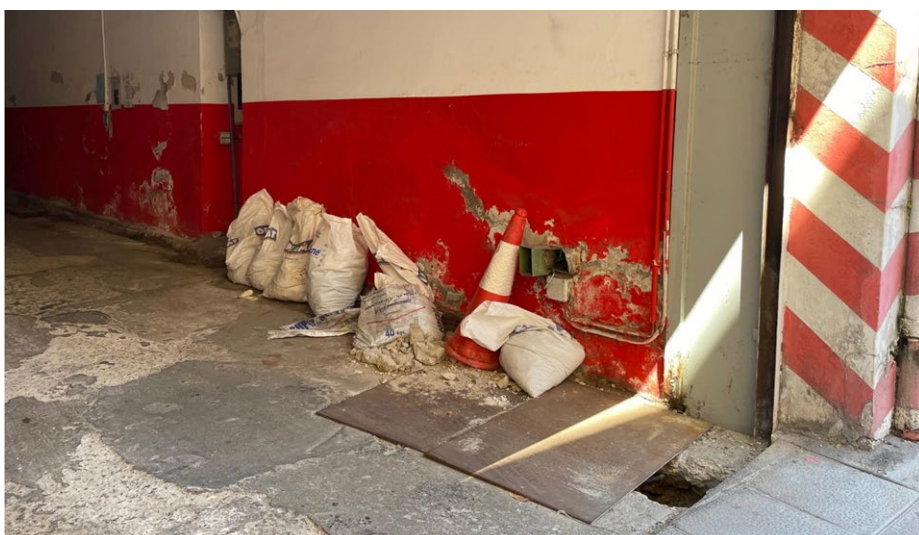
FIGURE R1.7. Presence of dampness in buildings
